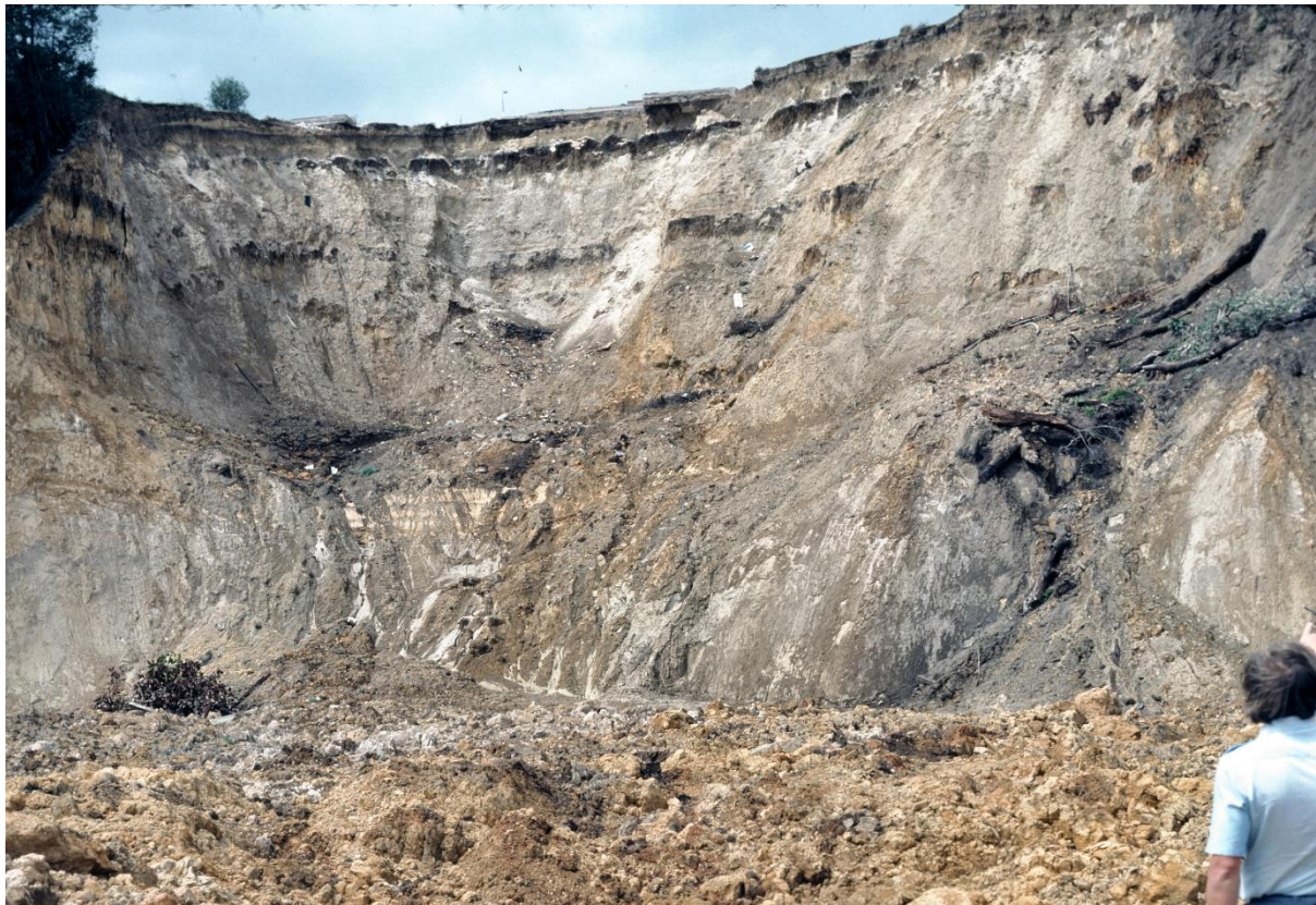
Fig. 3. Landslide at Bramley Drive, Omokoroa, photographed in October 1979, barely two months after the initial main failure event on 9 August that year. The landslide, ~60 m across, had a run out distance of at least 150 m from the base of the slope; the cliff edge receded by ~20 m, forcing the eventual removal of five houses in close proximity to the main scarp (Gulliver and Houghton, 1980; Moon, 2016). The slide was reactivated in May 2011 and in April and August 2012, causing further regression of the scarp. Photo: D.J. Lowe.
